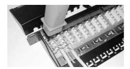
Press foil or braid shield to contact ground, and keep the cable straight.
